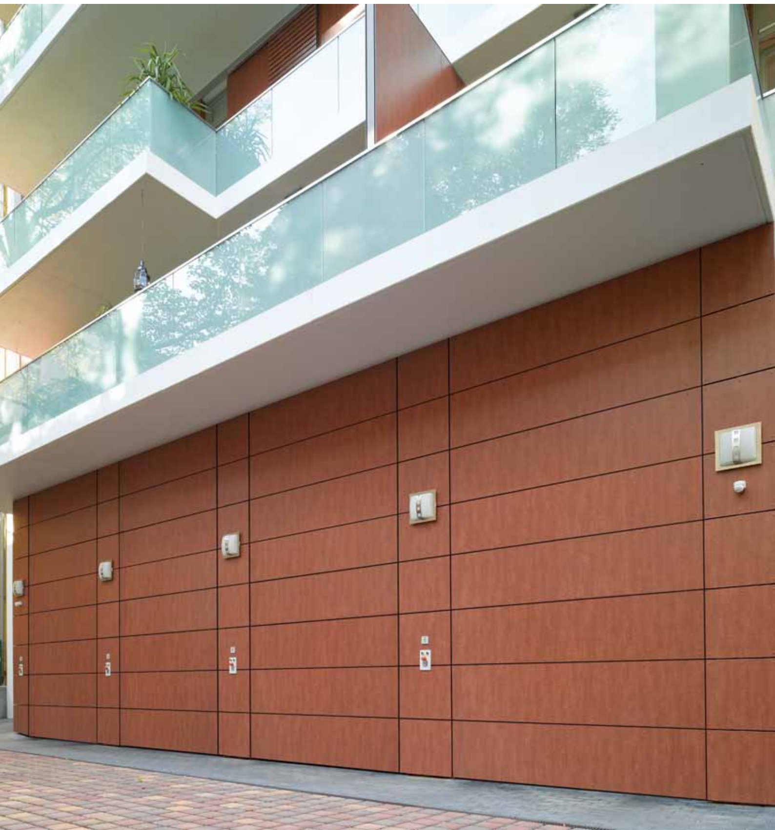
On-site cladding with laminated timber boards
